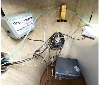
GEO-Inspector was hired to install the monitoring equipment, collect daily readings, and present the data to the client on its custom visualisation platform.
